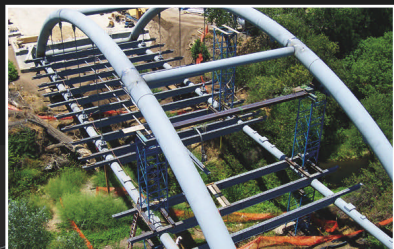
Lewis Avenue Tied Arch Truss Bridge - Vehicular Bridge 42" x 3/4" wall pipe cold bend with no deformation (107'-4 1/4" CLR)
