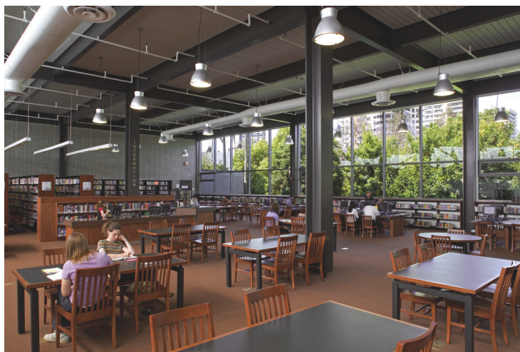
All exposed steel in the library meets AISC's AESS requirements.
